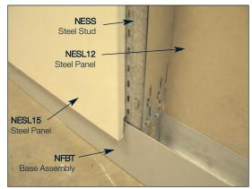
the Element until it pushes back over the hook-lugs to hit the Steel Stud face. The Element can now be pulled down over the hook-lugs.
