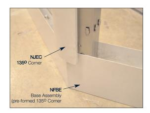
**Note:** When sliding the 135° Corner Post along the Head and Base Tracks and around the elbow be careful not to scratch the Head and Base Tracks. Two people - one person at the top and one at the bottom - should do this together.
