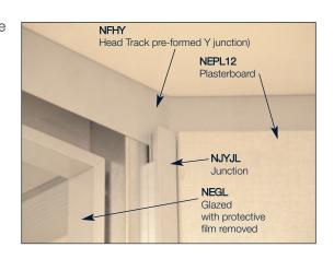
6.6 The joint gap between two adjacent Glazed Elements is the standard 4mm.
